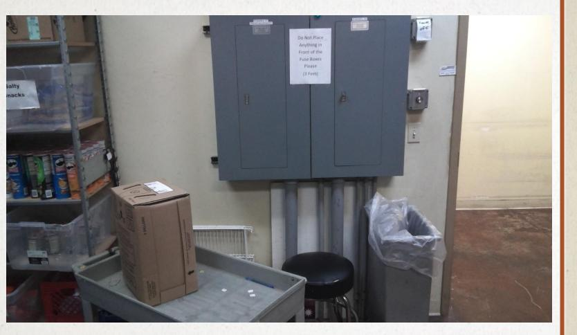
A working space of not less than 30 inches (762 mm) in width, 36 inches (914 mm) in depth and 78 inches (1981 mm) in height shall be provided in front of electrical service equipment. Where the electrical service equipment is wider than 30 inches (762 mm), the working space shall be not less than the width of the equipment.
